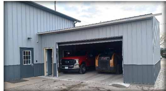
Public Works garage addition
